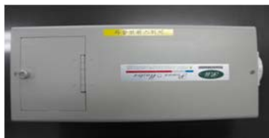
Diagram 3-21 ATS, Auto Transfer Switch
